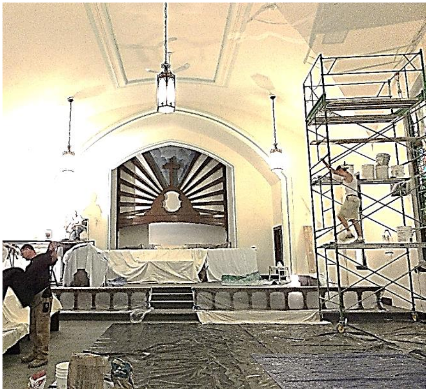
Plasterers needed ladders and scaffolding to reach all of the places needing repair.
