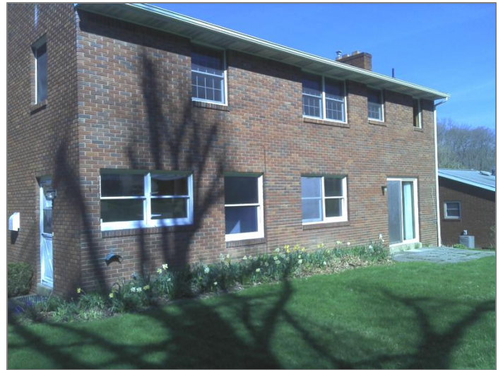
2. At the back, the windows on the first floor are the old ones. New windows have been installed on the second floor. (The trustees will replace the sliding glass door later this year.)
