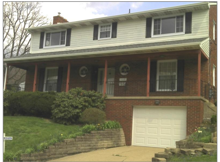
4. The project is complete and all 22 windows have been replaced.
